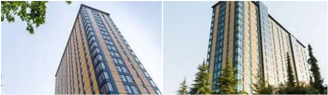
Fig. 3. 18 story Tallwood Brock Commons in Vancouver: Made naturally from wood
