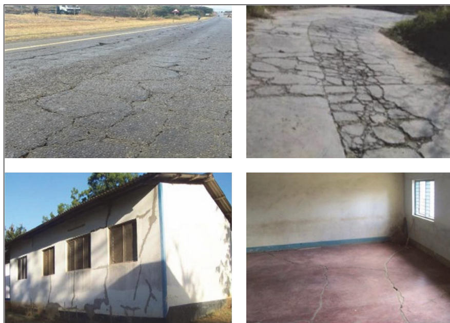
FIGURE 3: Typical representation of geotechnical constructions founded on black cotton soil (BCS) in Shire Valley.
