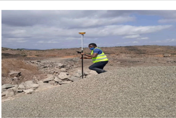
FIGURE 7 Recording elevation at different points of the stockpile.
